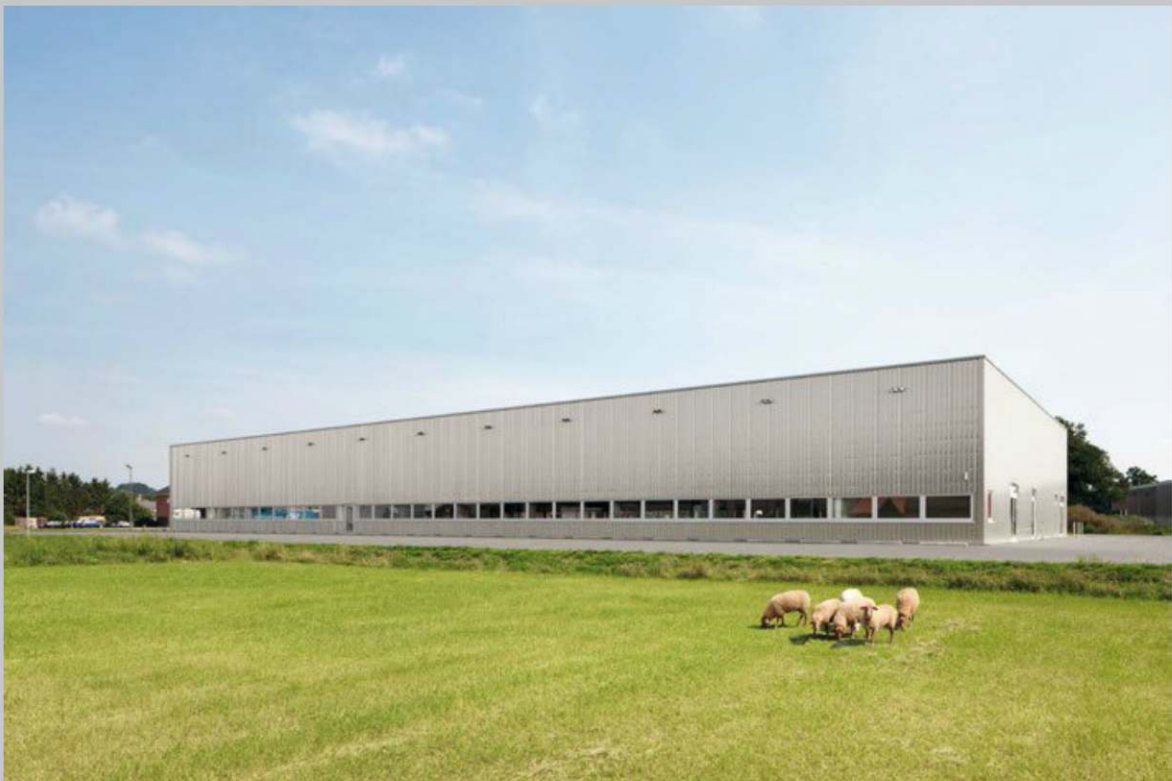
Fig. 2 – Entrepôt, Osnabrück. Photo: Marcus Bredt
